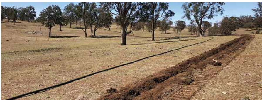
Below: 4km of pipe laid to fill troughs Right: 1 of 11 completed troughs Bottom right: Filling the new troughs
