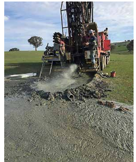
Bottom: New bore producing 19,000 litres an hour
